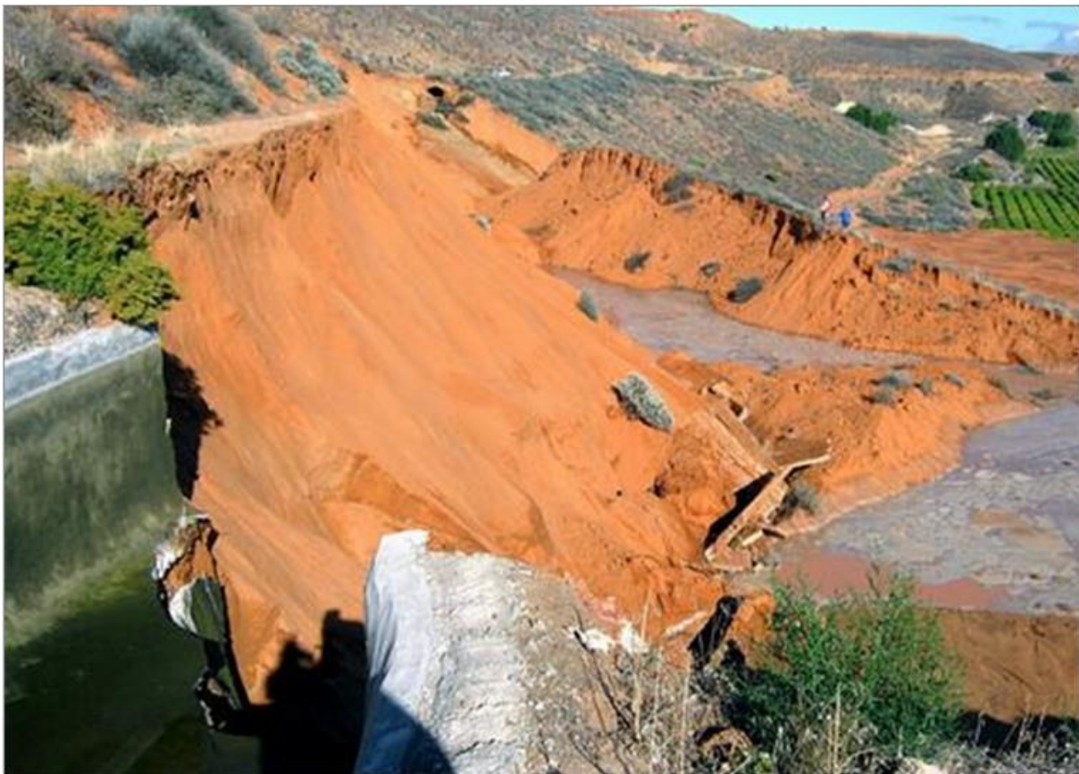
Figure 2-5: Lower Olifants Canal break in 2015
