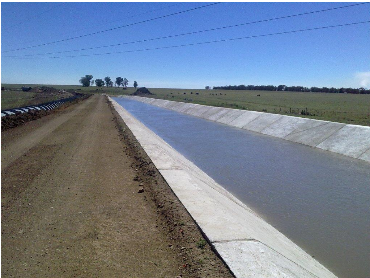
Figure 2-10: Vlakfontein Canal example of a new canal
