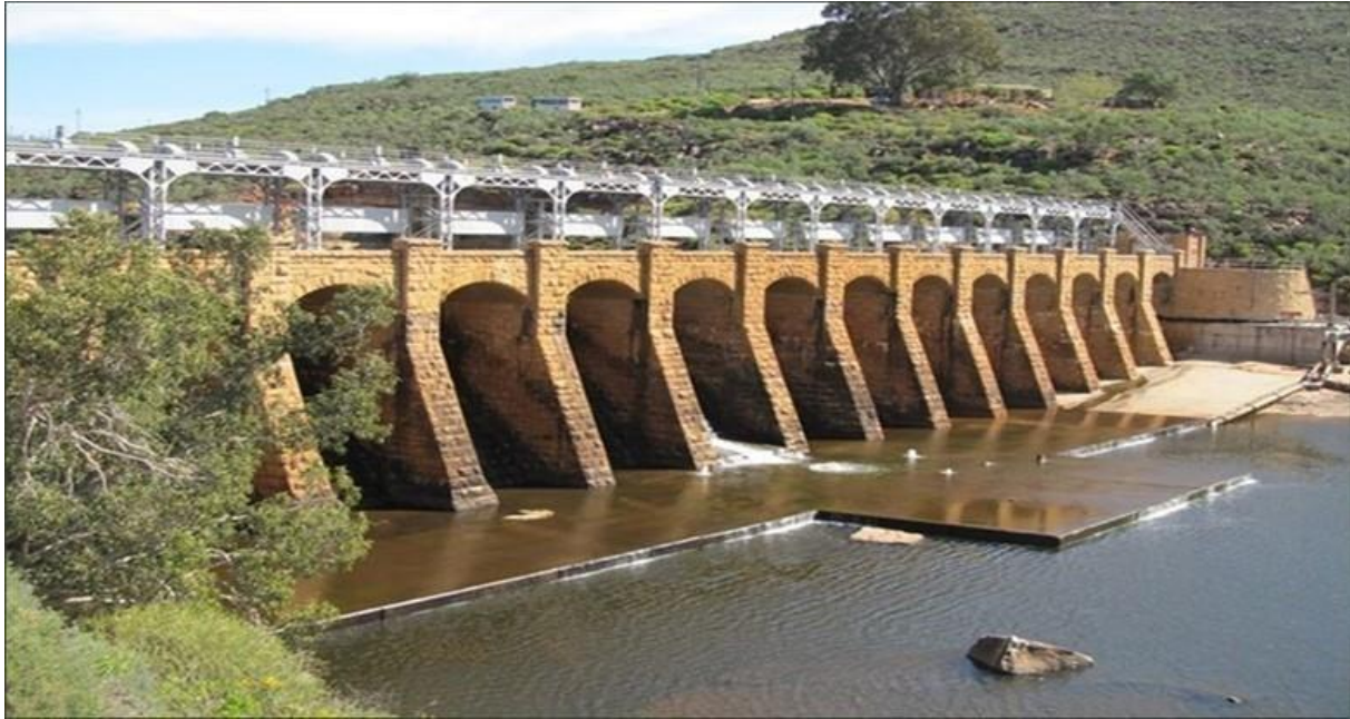
Figure 2-3: Concrete masonry Bulshoek Weir
